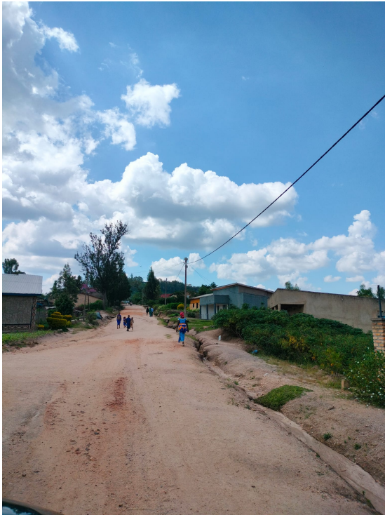
(a) Unpaved road
